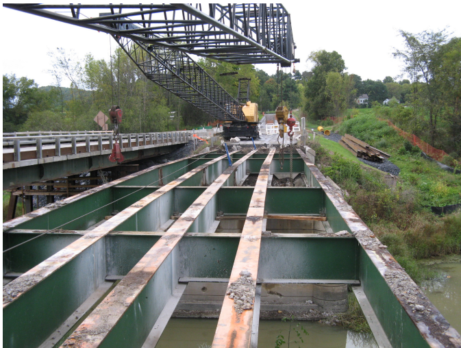
Decking (what was left of it) removed from the 1938 bridge.
