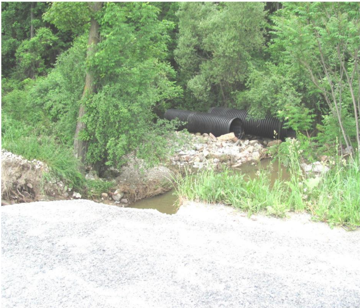
A shot from Clark Road where the culverts washed out and took a ride in the May 29 th storm.
