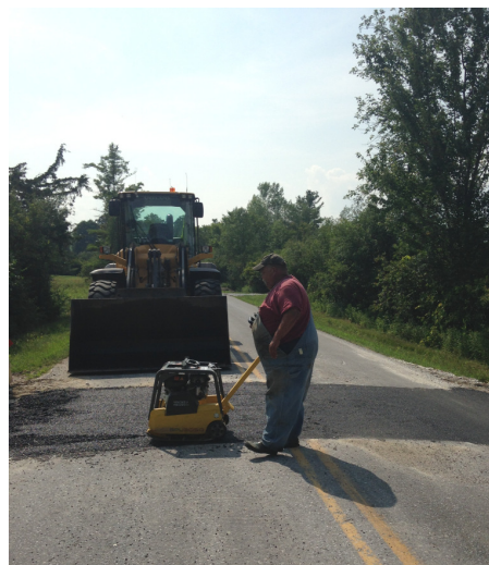
Compacting the West St Culvert
