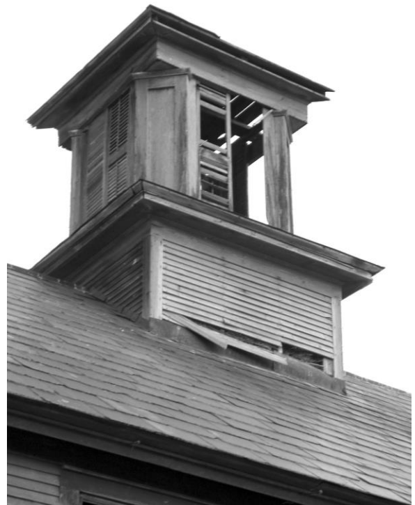
Cupola on 19th century barn.
