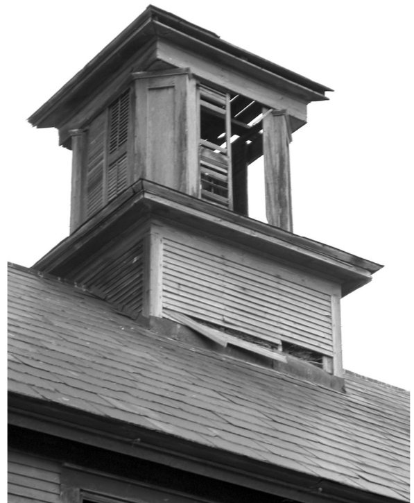
Cupola on 19th century barn.
